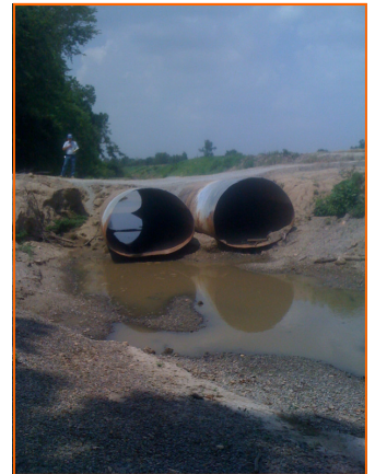
Flooding damaged crossing on County Road 274 near Randles
