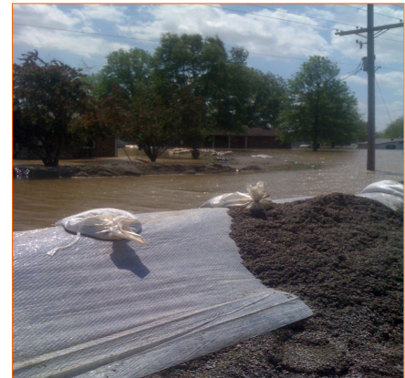
Emergency levee constructed for the 2011 flood.
